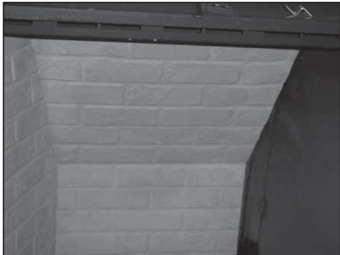
Figure 15.3 Install Upper Back Refractory
